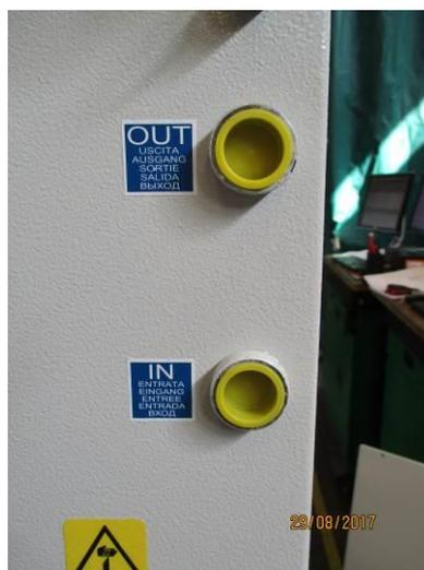
Picture 4 –Hydraulic connection plate
